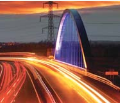
Toombe Bridge: DRD Roads Service
