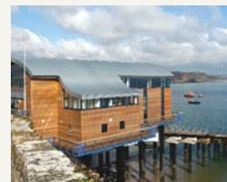
RNLI Lifeboat Station Tenby: Dean & Dyball Construction Ltd
