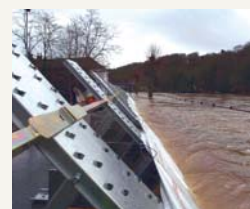
Temporary flood defence at Ironbridge
