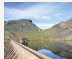
Stwlan Dam: First Hydro Ltd
